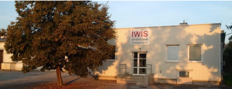
Plant Strakonice, Czech Republic
