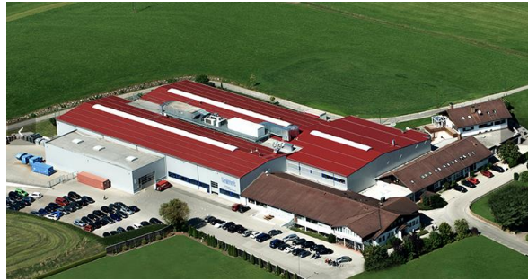
Plant Rieden, Germany
