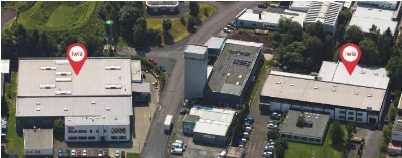
Plant Wilnsdorf, Germany
