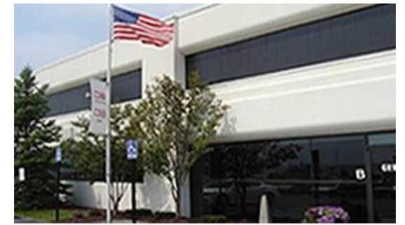
Plant Grand Rapids, USA
