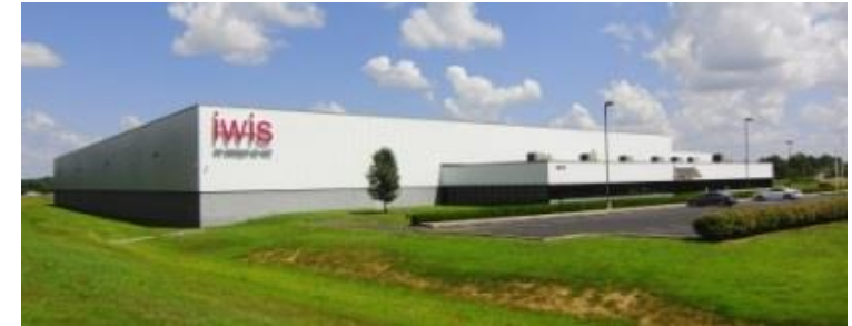
Plant Murray, USA
