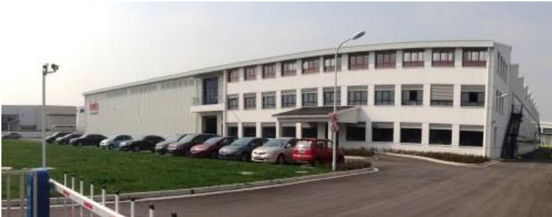
Plant Suzhou, China
